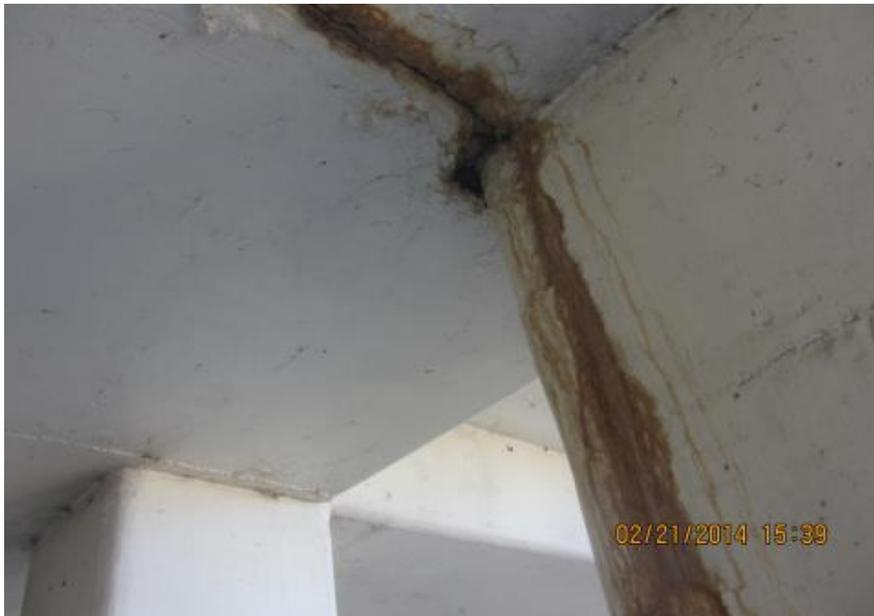
*Seismic expansion joint with leak from roof*
